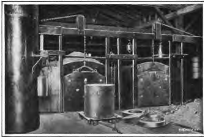
Fig. 16. Pot Annealing Furnace, showing Pot just drawn out
